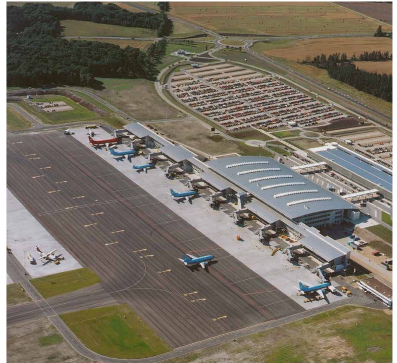
Densiphalt® on aprons and taxiways.
