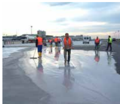
Installation of Densiphalt®.
