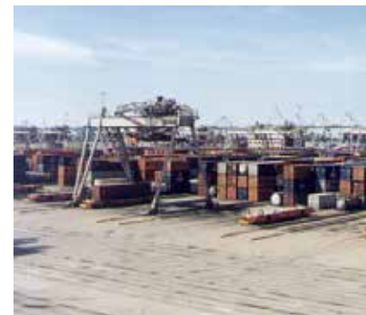
Container handling on Densiphalt® pavement.
