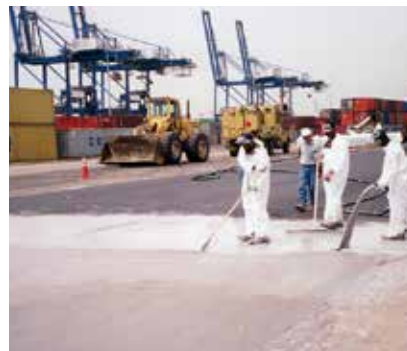
Installation of Densiphalt® mortar.
